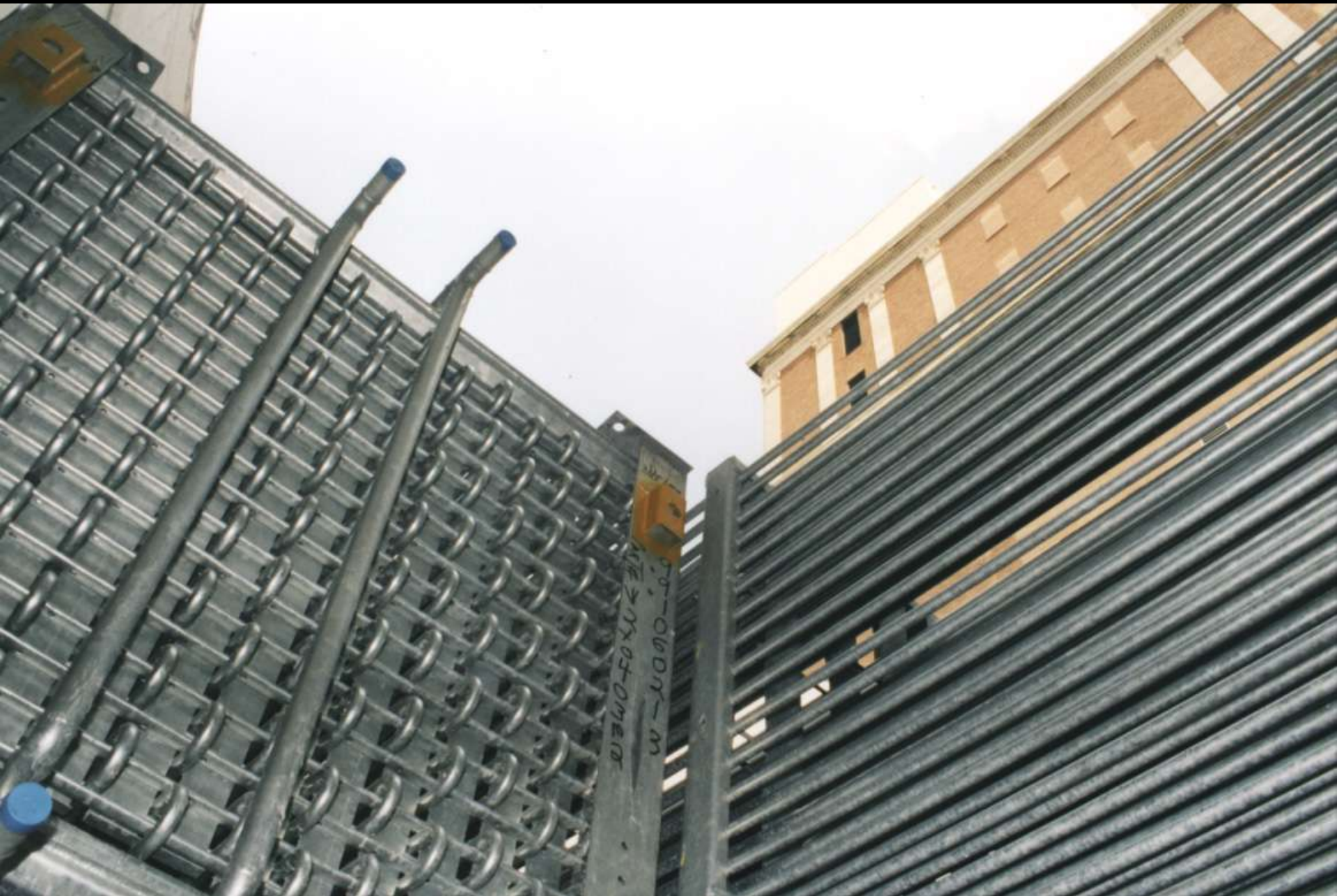
Comfort Link Market Center Chilling Station – Construction (1999)
