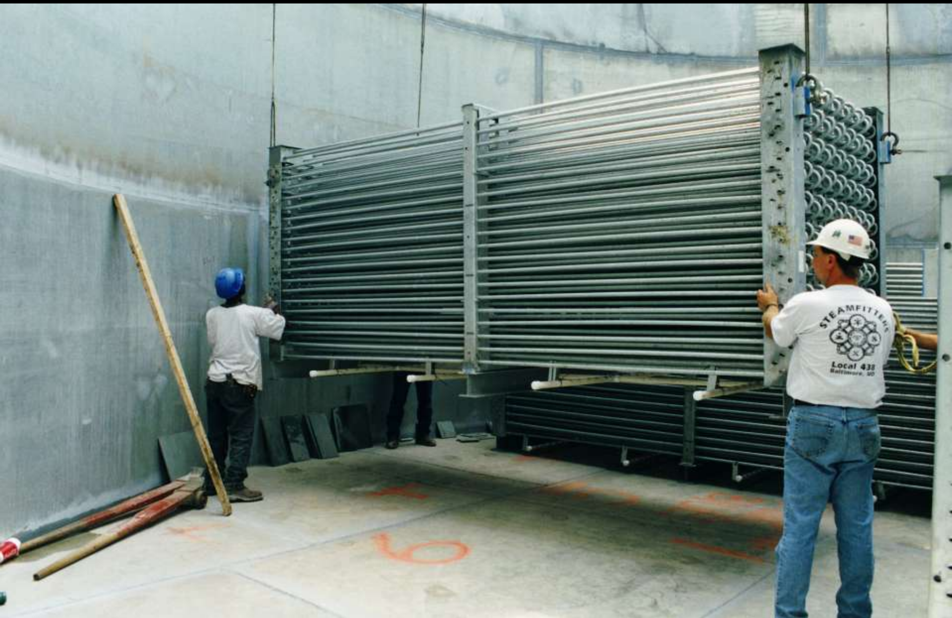
Comfort Link Market Center Chilling Station – Construction (1999)
