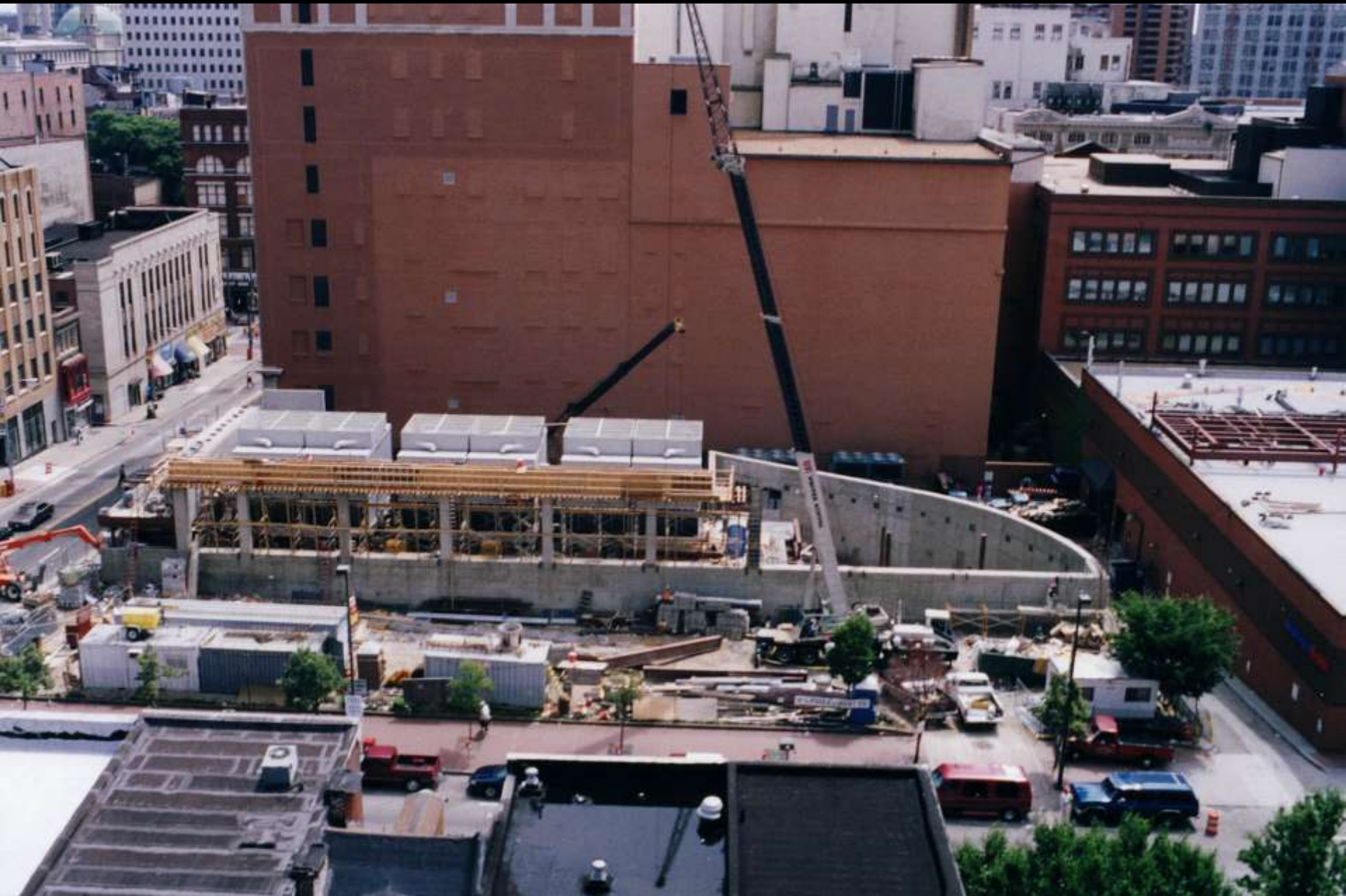
Comfort Link Market Center Chilling Station – Construction (1999)
