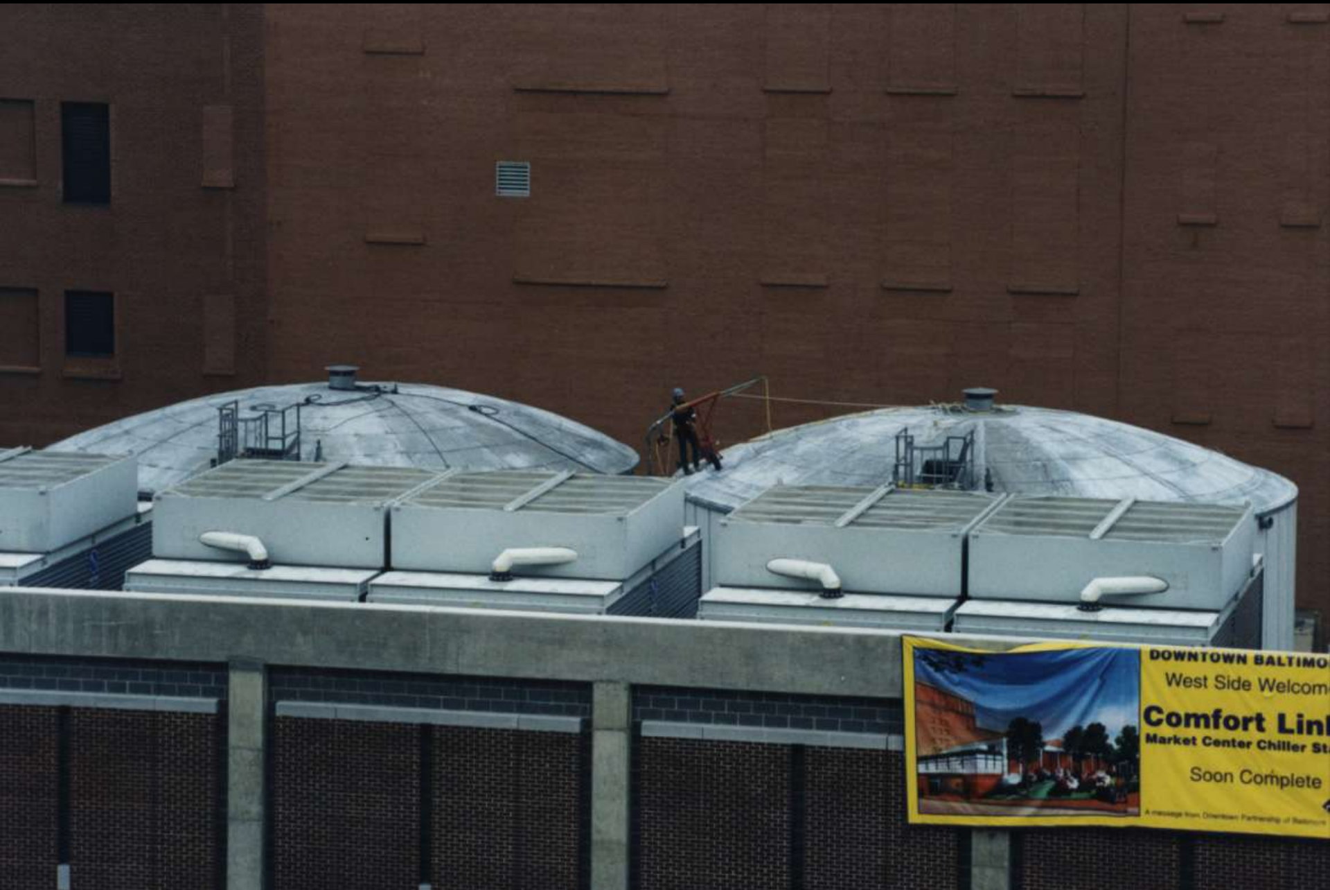
Comfort Link Market Center Chilling Station – Construction (1999)
