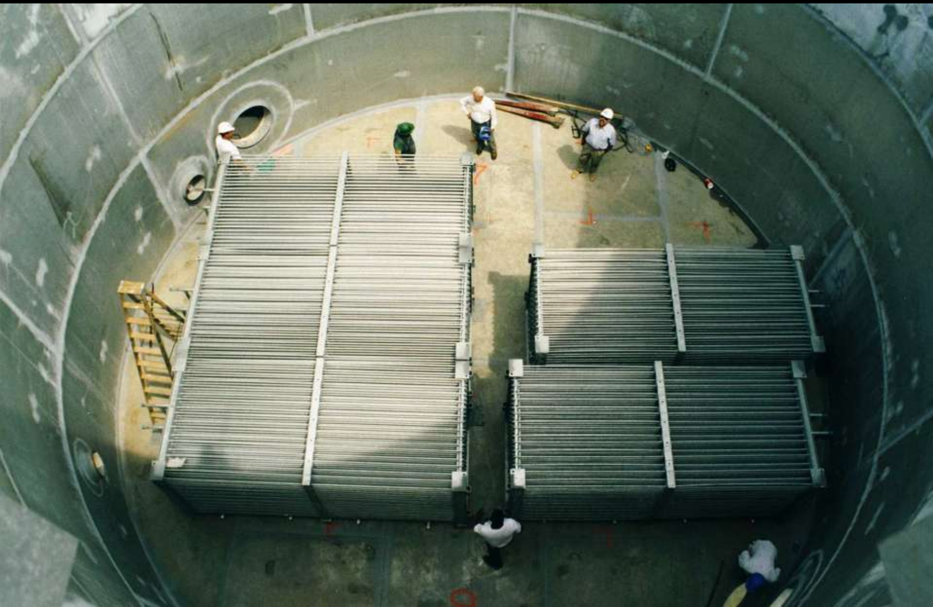
Comfort Link Market Center Chilling Station – Construction (1999)
