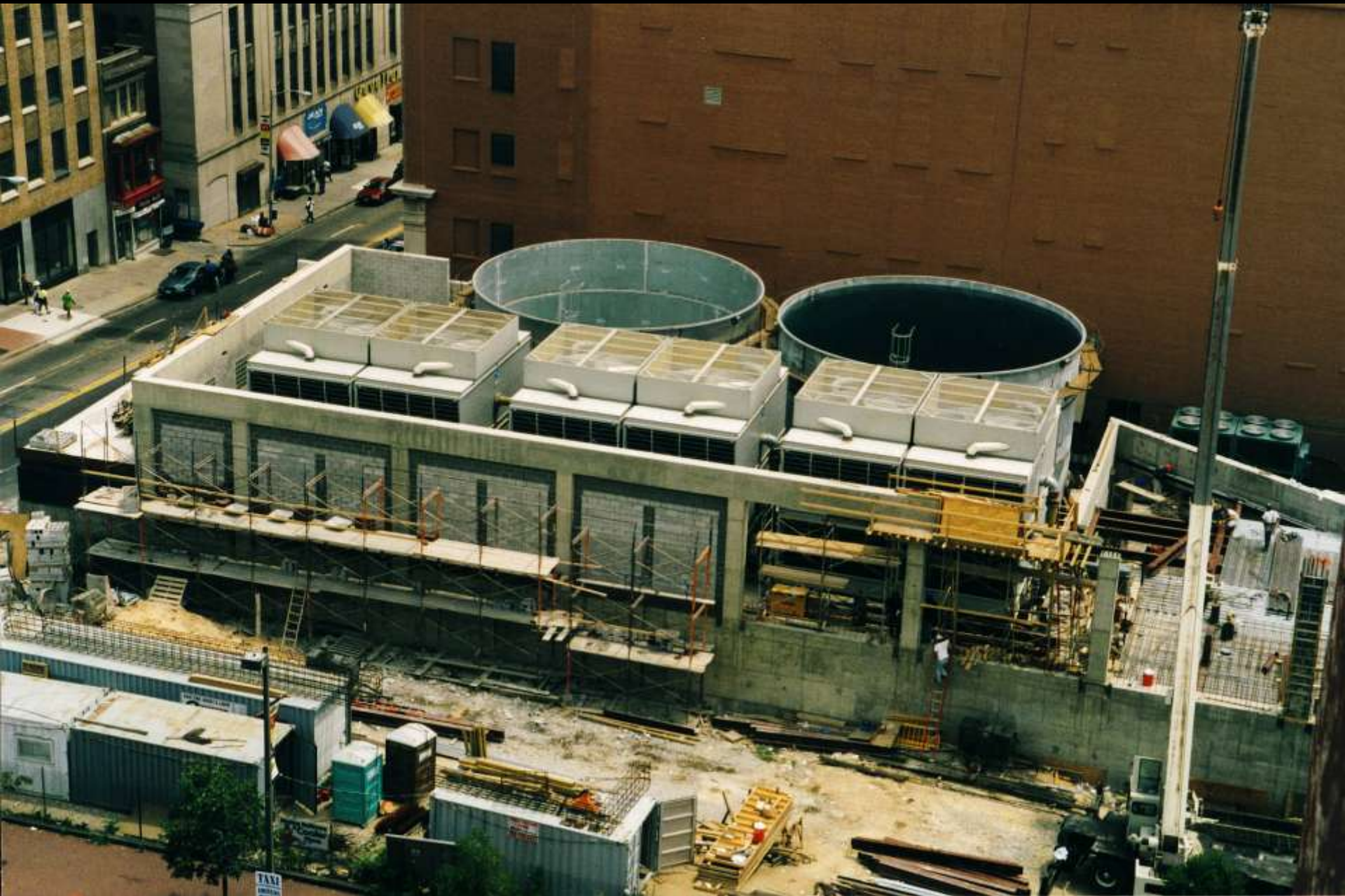
Comfort Link Market Center Chilling Station – Construction (1999)
